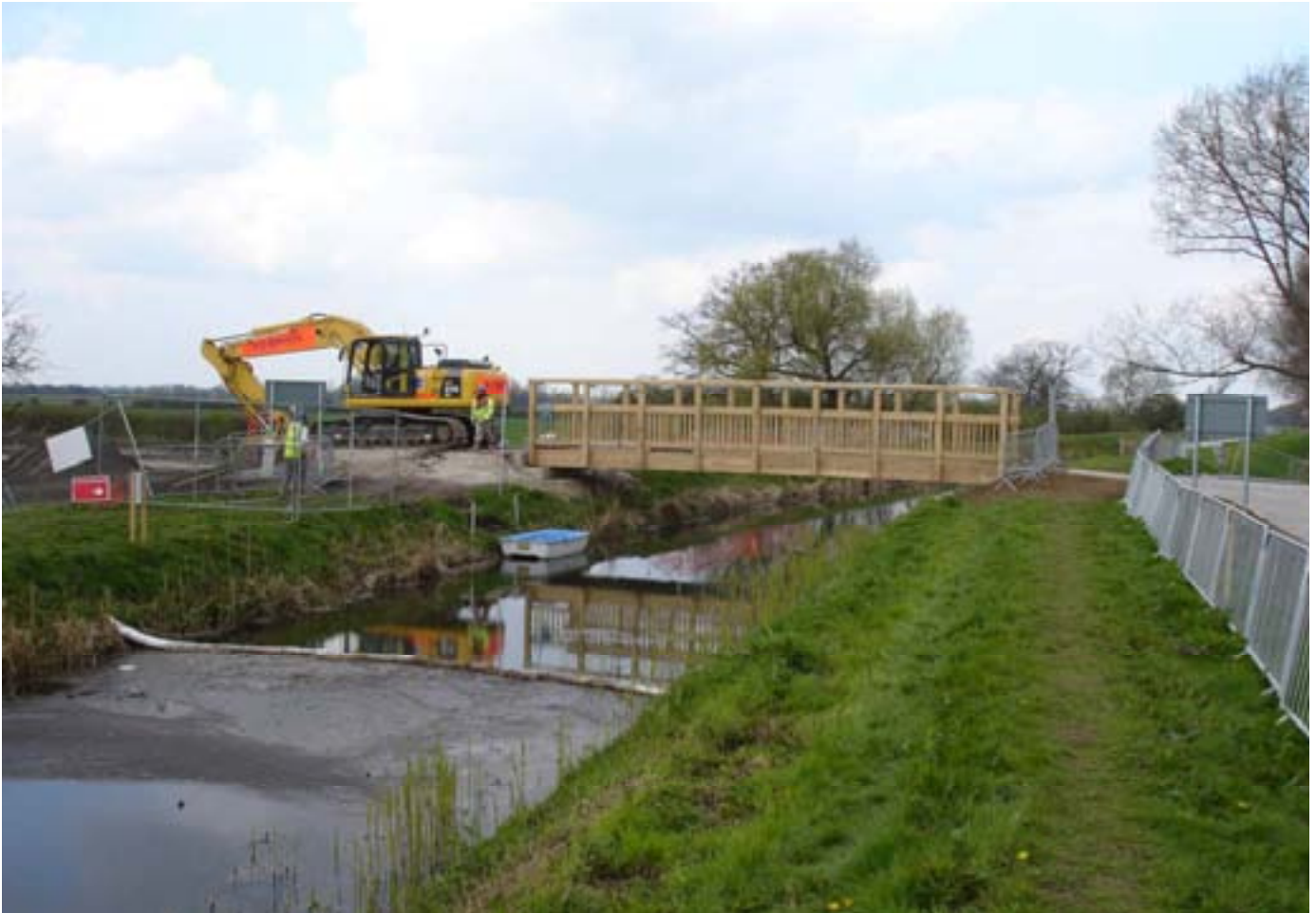
Swaffham Bulbeck Lode Bridge being moved into position
